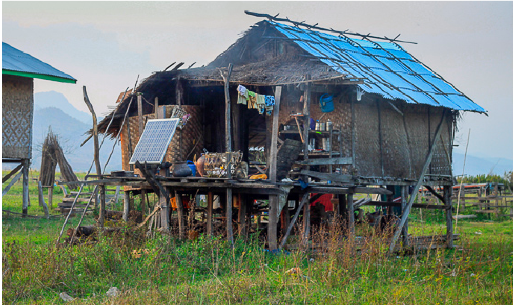
Than Bayar Khon village, Myanmar. Solar PV installed by Global Environmental Institute, Beijing.
